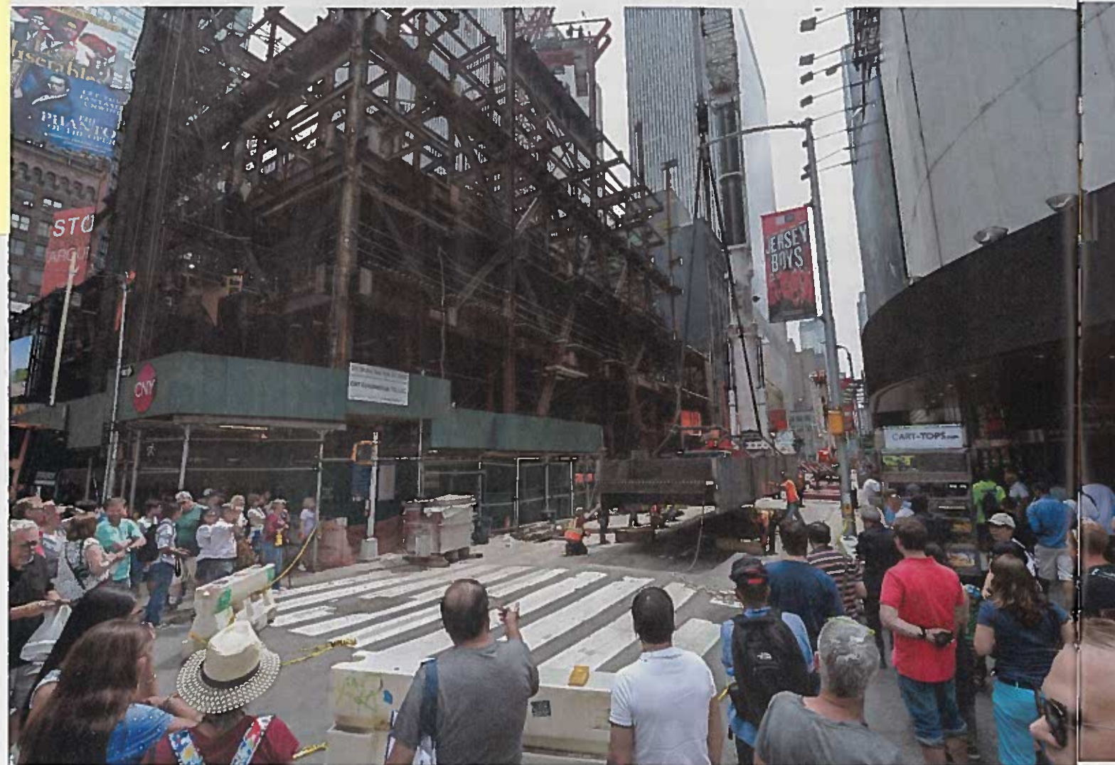
GIRDER GAWKERS The fishbowl project in the heart of Times Square attracted crowds of onlookers every time there was a big pick, such as this 60-ton girder.
