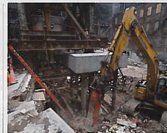
FLEETING FOUNDATION Stripped old steel was supported by an elaborate shoring system bearing on caisson clusters.
